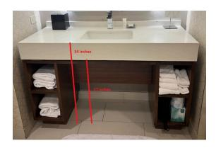
The water controls are handoperated, can be operated with one hand, do not require tight grasping, pinching and twisting of the wrist
