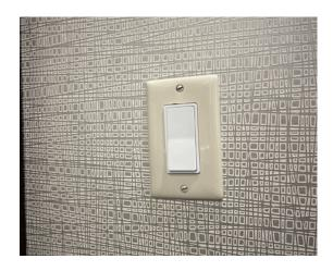
The switches in the room are hand-operated and have a large push plate located at a height of 47 inches from the floor
