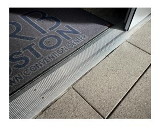
The door threshold height is minimized with a large transition plate, creating a nearly flat entry
