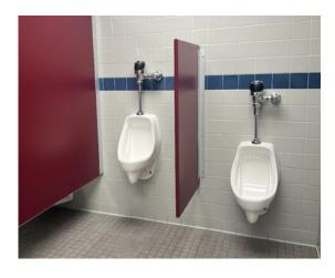
The urinals are installed at two heights, 16 inches and 24 inches, with a clear floor space of over 60 by 60 inches in front of each
