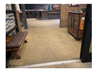
The door threshold height is minimized with a large transition plate, creating a nearly flat entry
